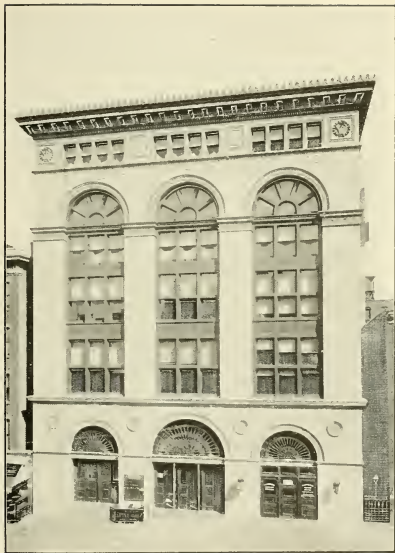
ST. BARTHOLOMEW'S PARISH HOUSE—205 East Forty-second Street.
